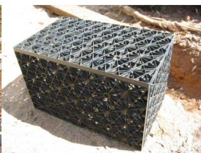
CSAT Marshall Greywater Reuse System collects water in a tank, pumps it through a series of pipelines and disperses water through Atlantis cells.
