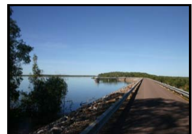
Darwin River Dam- Darwin Drinking Water Supply
