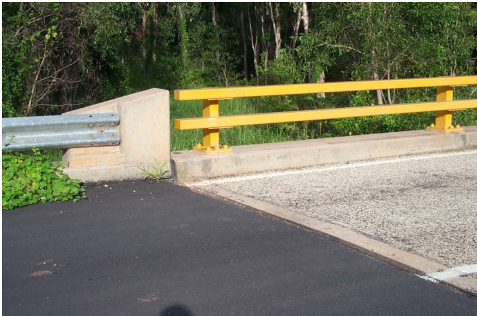
Photo 12 Example of Bench Mark on bridge abutment
