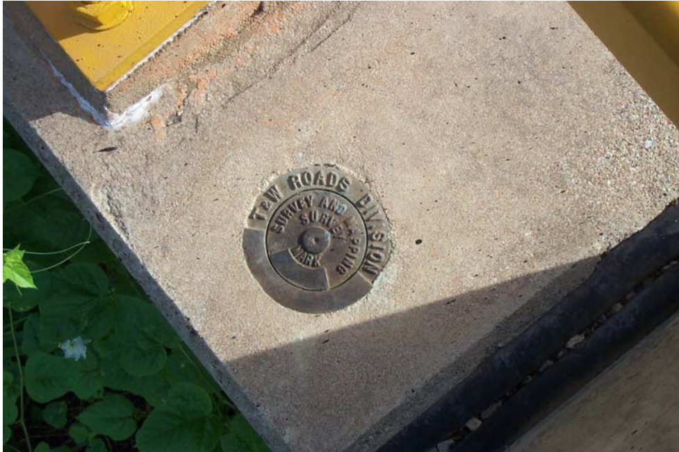
Photo 11 Example of Bench Mark on bridge abutment
