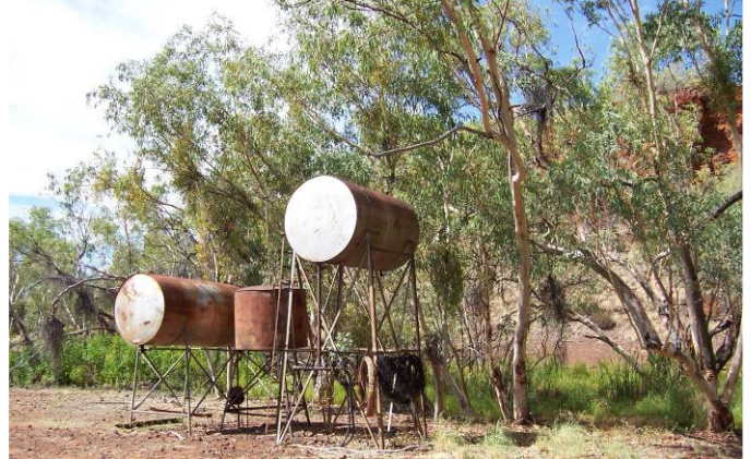
Photo 1- Unsatisfactory Fuel Storage
