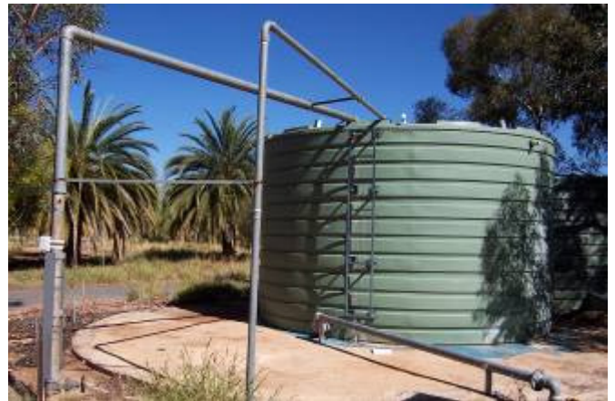
Another effective form of backflow prevention is to utilise a break tank that has an air gap to ensure contamination of the resource can not occur.
