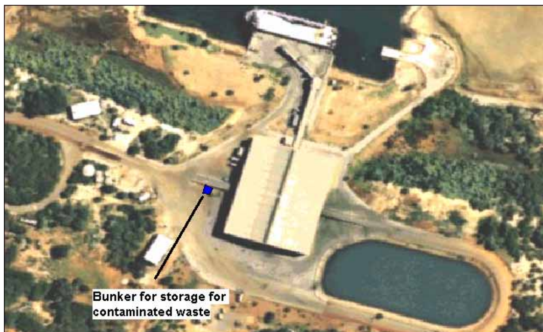
Figure 2. Contaminated waste bunker at the Bing Bong Loading Facility
