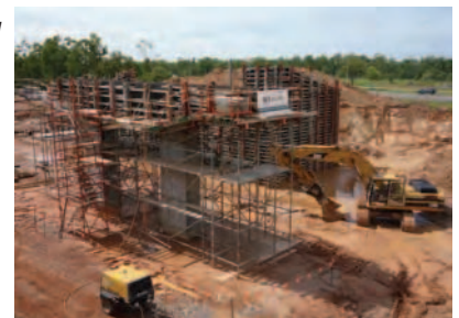
Left: Formwork around one of the headstocks before the concrete is poured. This structure will support the bridge carrying outbound traffic.
