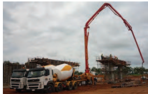
Left: Formwork around one of the headstocks before the concrete is poured. This structure will support the bridge carrying outbound traffic.
