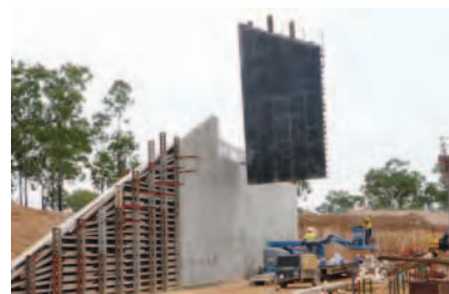
Left: Concrete formwork underway on the Northbound bridge.
