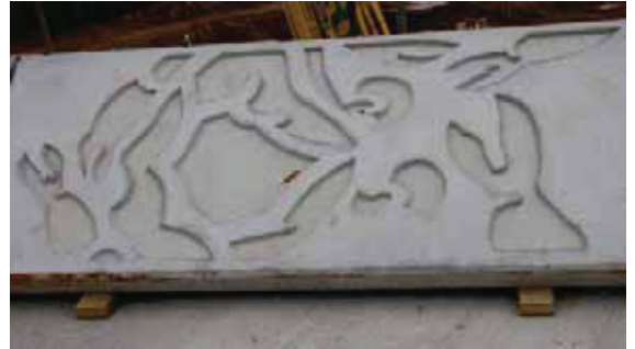
Above: A precast concrete parapet featuring crabs for the bridge closer to Darwin City.
