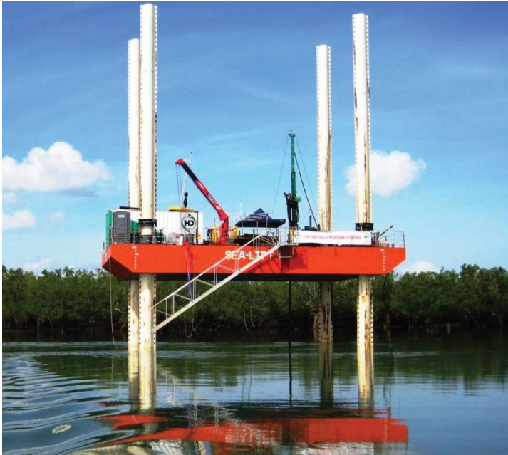
Jack-up barges similar to these will undertake the drilling activities. The barge is 25m long and 10m wide.
