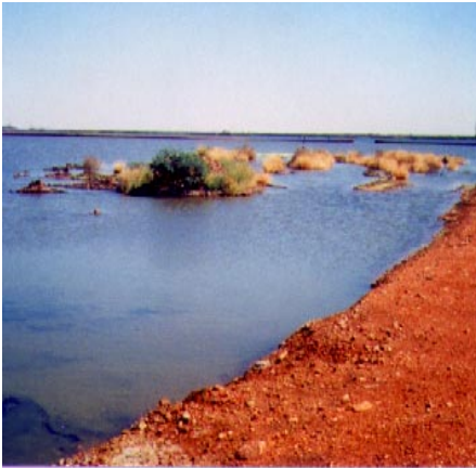
Avoid the formation of islands and other roosting features within tailings storage facilities.
