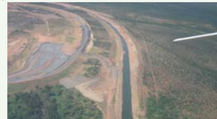
The above photograph shows the upstream end of the McArthur River Diversion, and the cut off section of the old McArthur River channel to the bottom left. During times of flood, water passes overland between the two.
