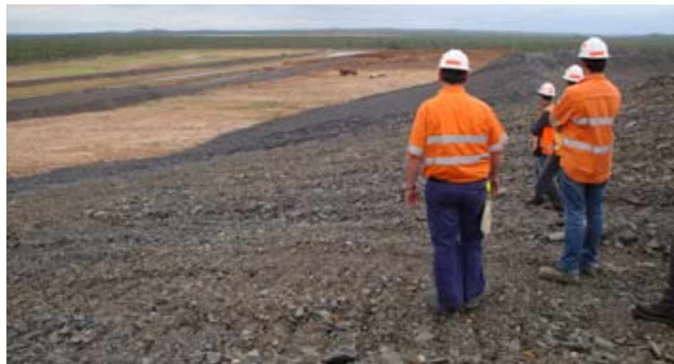
The Independent Monitor team inspected the progress of the Overburden Emplacement Facility in May 2010. The OEF receives waste rock or 'overburden' from the mine pit. Some of the waste rock has the potential to form acid if it is exposed to water and air, so the proper placement of 'potentially acid-forming' and 'non-acid forming' rocks is essential to avoid environmental damage from releasing acid into the environment.
